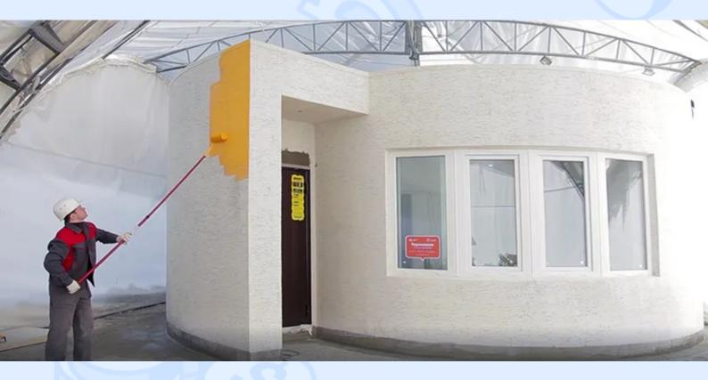
The first 3D printed house built completely on-site was brought to life by the Apis Cor 3D Construction company and Russian public developer PIK. The building looks like a normal one-storey cottage with an unusual design - the house is in the shape of a rotor. It was made from a concrete mixture topped with a weather-resistant roof. 3D printing had been utilised for house manufacturing before, but houses had been built in pieces, which were later brought together as a single building.
